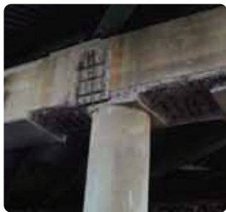
Overhead/ Vertical Repair
