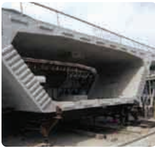
High Performance Concrete
