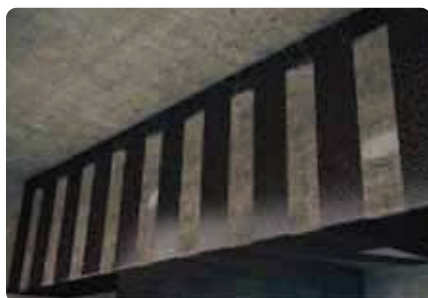
FRP structural strengthening
